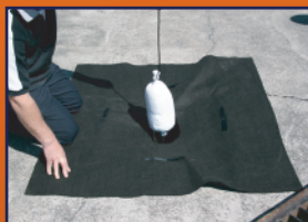
2. Lay Bilge Sock in place.
