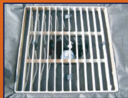
3. Attach sock to grate and fasten velcro.
