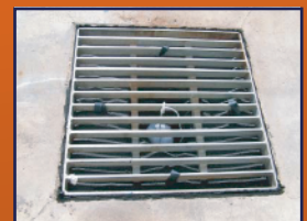
5. Drain Filter is now in place.
